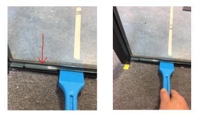
**2-9.** Have the glass strip to the top ready, click it firmly in the groove and install wedge rubber in the profile to lock the glass strip with. Proceed with the assembly of all glasses.
