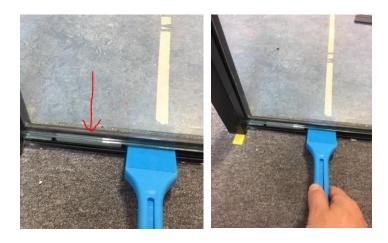
Have the glass strip to the top ready, click it firmly in the groove and install any wedge rubber in the profile to lock the glass strip. Proceed with the assembly of all glasses. (The glass moldings are recommended to be cut off bluntly. (90-degree angle)
